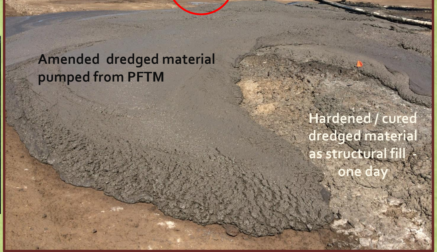
Pneumatic Tube Mixing for Contaminated Soft Sediments
