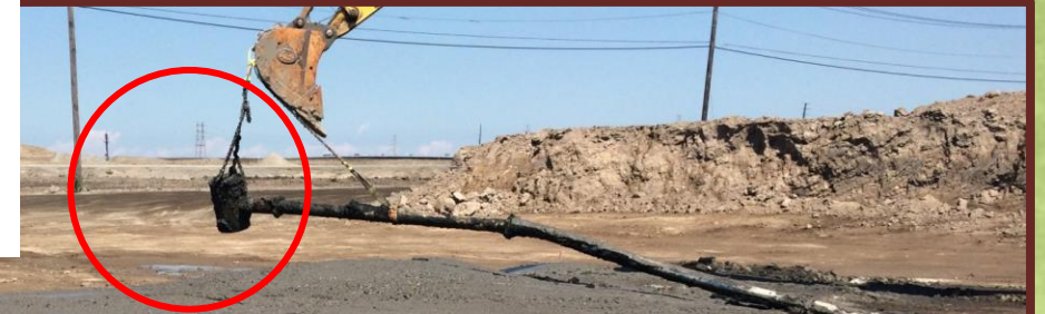
Pneumatic Tube Mixing for Contaminated Soft Sediments
