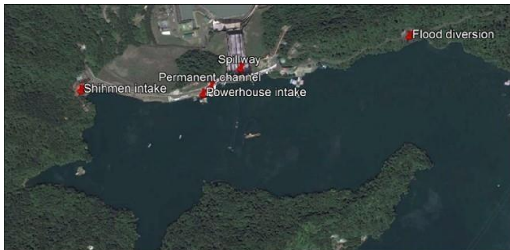
Figure 5-3 Location of existing outlets that may be used for sediment release (Google Earth image)
