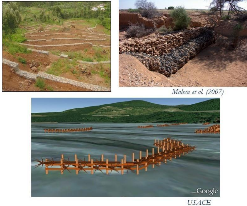
Figure 3-33 Some examples of (soft-structural) catchment and river sediment management measures
