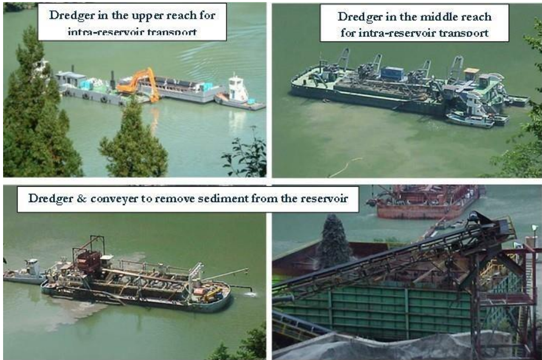
Figure 5-8 Sediment dredging and removal arrangement (provided by J-Power)
