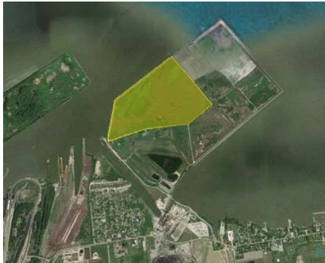
Figure 3-29 One of the Great Lake CDFs (extended in 1994) at Toledo harbour - Island 18
