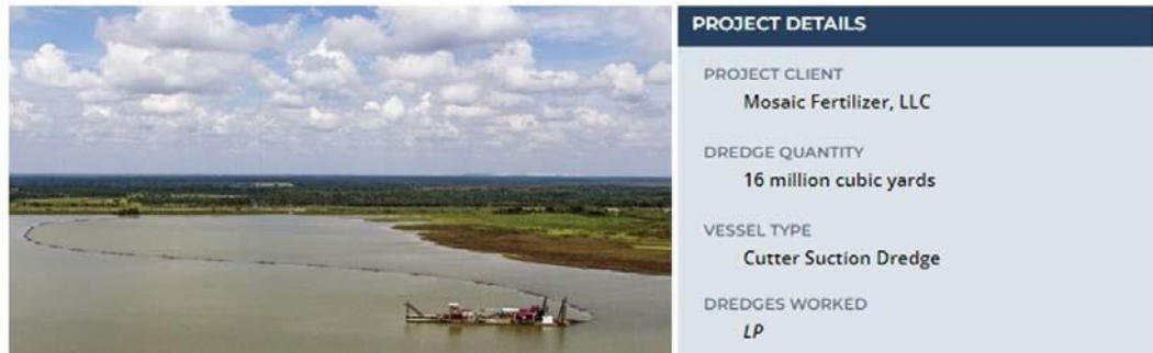
Figure 5-26 Dredging operation at Mosaic (left) and the project details (Great Lakes Dredge & Dock Company)
